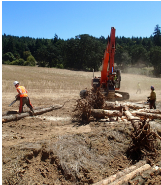
from top: Initial conditions; Installing large woody debris
