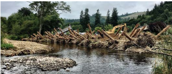
top: Initial conditions; above: During construction
