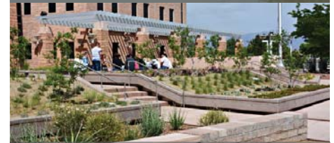
Capturing rainwater for reuse reduces potable water use by 75%+ at federal courthouse, Albuquerque, NM
