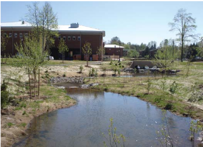
top: Initial conditions; above: Immediately after construction
