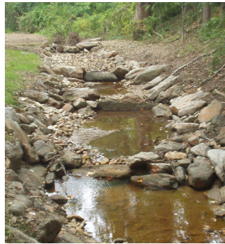
top: After construction – meandering stream connected to floodplain
