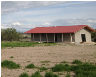
Straw bale house designed and built by students
