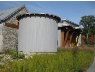
from top, clockwise: Constructed wetland for wastewater treatment; Rainwater treatment system made visible for education; 10,000 gallon cistern for harvested rainwater
