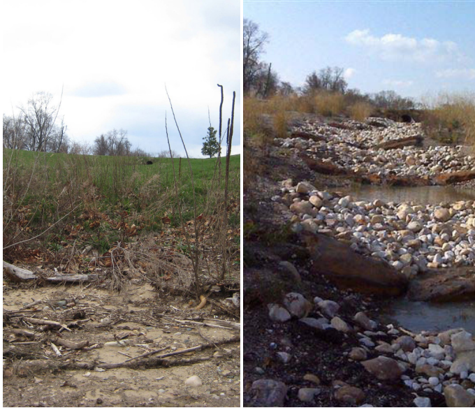
From left: Before and after construction
