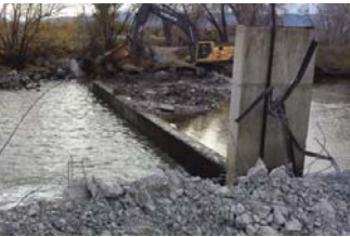
from top: River after dam removal; Removal of the dam
