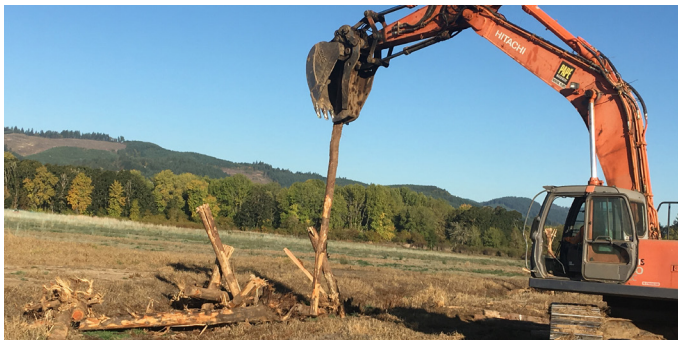
A log jam being installed.
