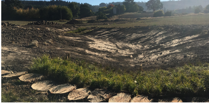
Looking up towards the new channel with grade control structures installed.
