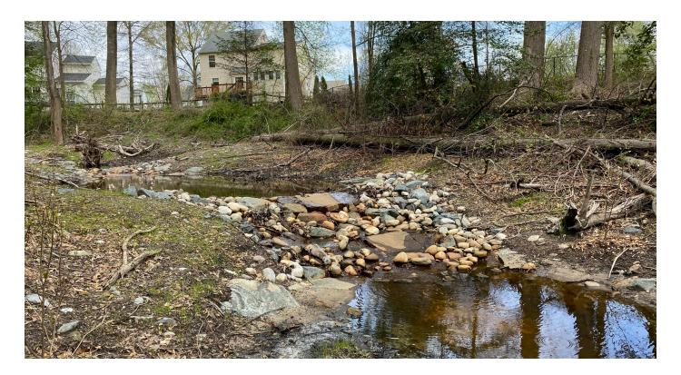
A degraded Coastal Plain outfall system was restored to enhance aquatic habitat, augment ecological function, and arrest erosional processes that would otherwise export sediment into the Chesapeake Bay.
