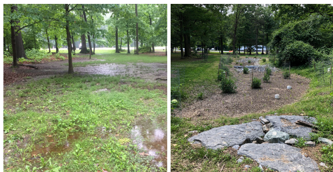
from top: Stormwater BMP captures runoff from parking lot, before and after; Capturing runoff near main stadium entrance, before and after; Bioretention cells capture stormwater, before and after
