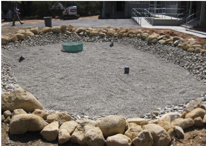
from top: State-of-the-art sea lion exhibit with underwater viewing wall; Newly built constructed wetlands before installation of vegetation
