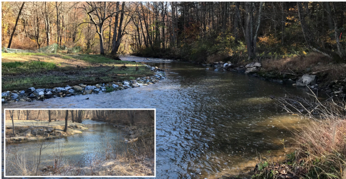
From top: Upper and Lower Gunpowder river before (inset) and after.
