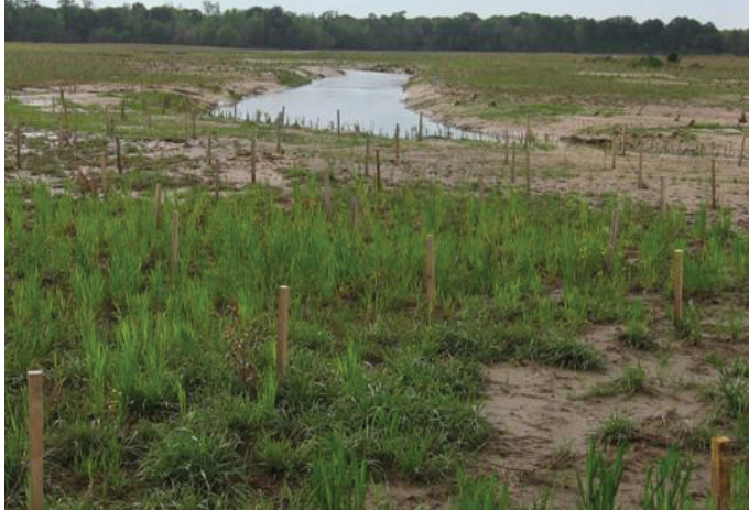
Remeandered channel one month after construction and planting
