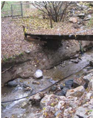
from top: After restoration; Initial conditions
