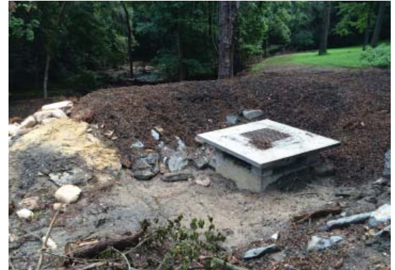
left: Outdated, failing storm drain system converted to a “bubbler” outfall leading to a natural system that filters water, adds habitat and recharges groundwater. above: Unlike the old outfall, which concentrated storm flows, the bubbler allows water to slowly “leak” into the stream and wetland treatment system.
