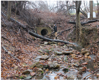
from top: the stream after restoration; before restoration
