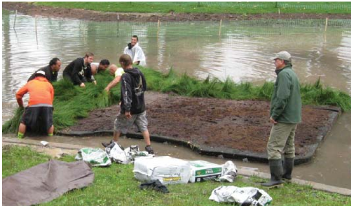
from top: Red Butte Creek at Miller Park after restoration with inset showing initial conditions; bottom: Liberty Lake Park and newly created wetland benches
