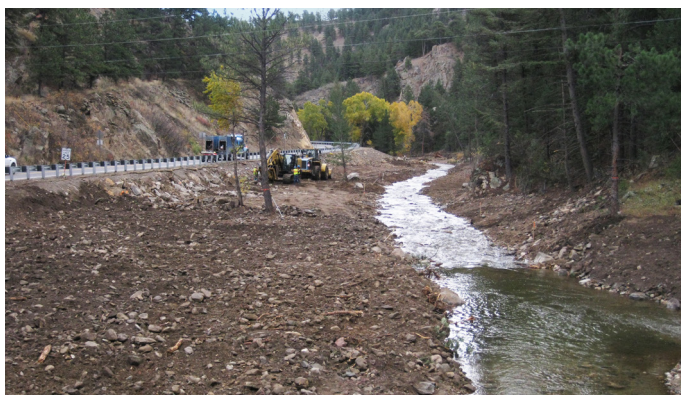
from top: Newly constructed road with stream before restoration; Immediately after stream relocation and floodplain creation; Coordinating construction of step pool
