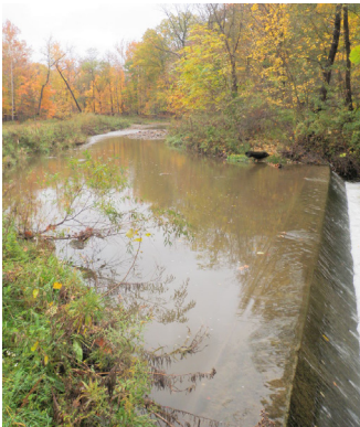
Initial conditions with bank erosion and large woody debris falling into stream (top) and lowhead dam to be modified to allow fish passage (bottom)
