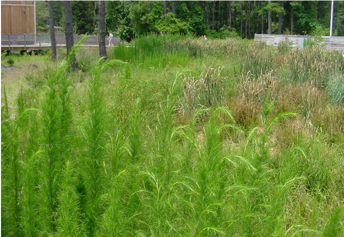
from top: Herbert H. Bateman Educational and Administrative Center; Constructed wastewater treatment wetland planted with native vegetation
