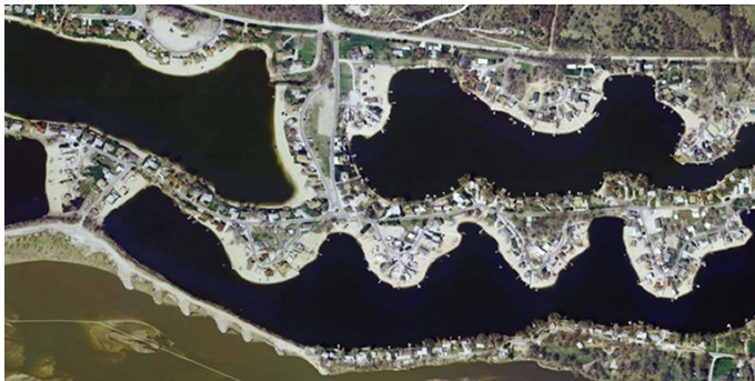
from top: Constructed wetland; Aerial view of the Hanson Lakes community
