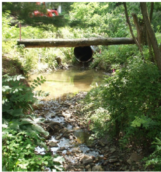
from top: After restoration; Before restoration—looking upstream at piped portion of first-order tributary before “daylighting,” relocating, and restoring the channel
