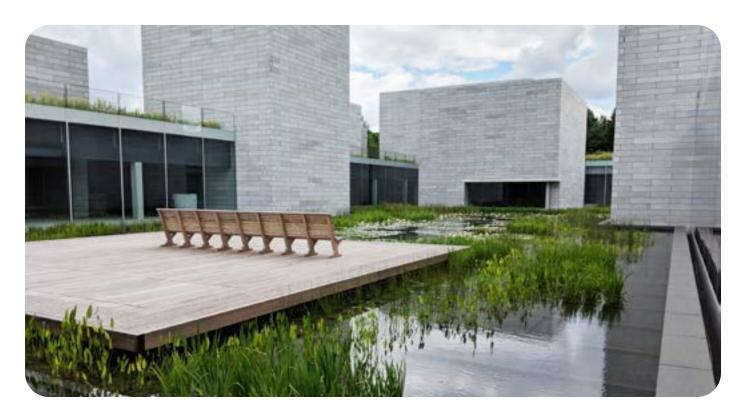
A museum's central water features meet the highly modern aesthetic while using a constructed wetland to biologically filter harvested rainwater from its rooftops.
