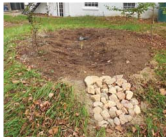
from top: Raincatcher planting plan; Raincatcher immediately after construction
