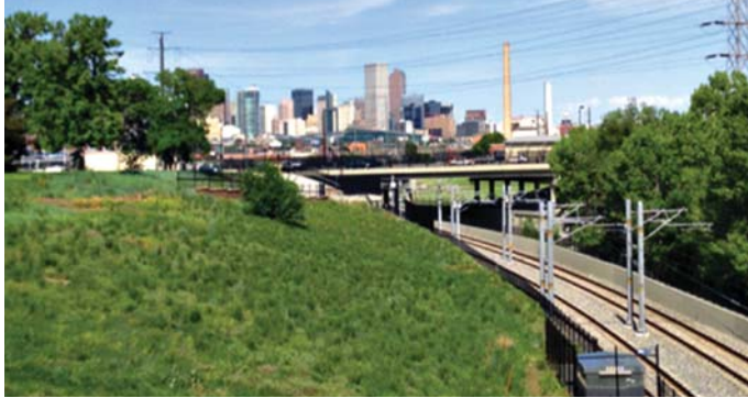
View of west Denver project area along light rail line
