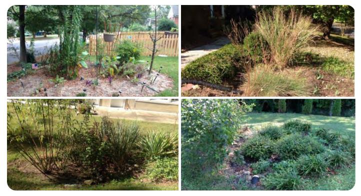
The project involved planting trees, disconnecting gutter downspouts, installing 108 cisterns, and constructing 42 bioretention SCM in residential lots to reduce nutrient concentrations in stormwater runoff.
