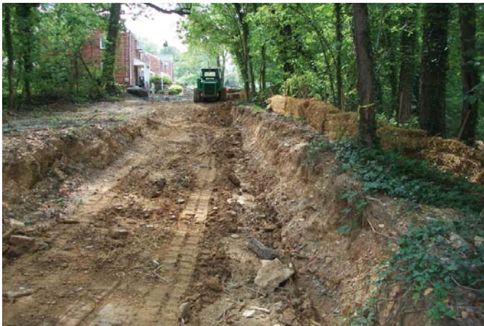
from top: Initial conditions; During construction
