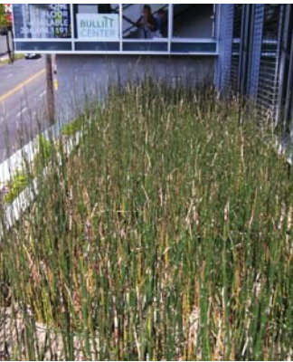
from top: A planted recirculating gravel filter provides treatment of all building greywater for reuse; Scouring rush ( Equisetum hyemale ) is planted throughout the gravel filter
