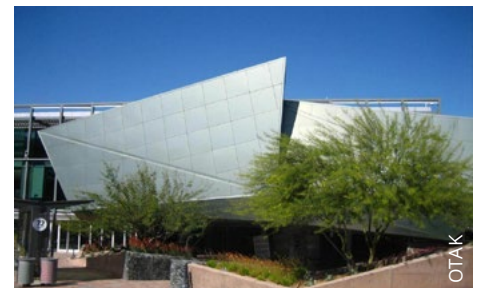
Tempe Transit Center
