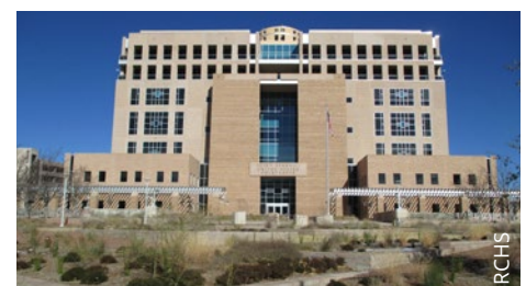
Pete H. Domenici Federal Courthouse
