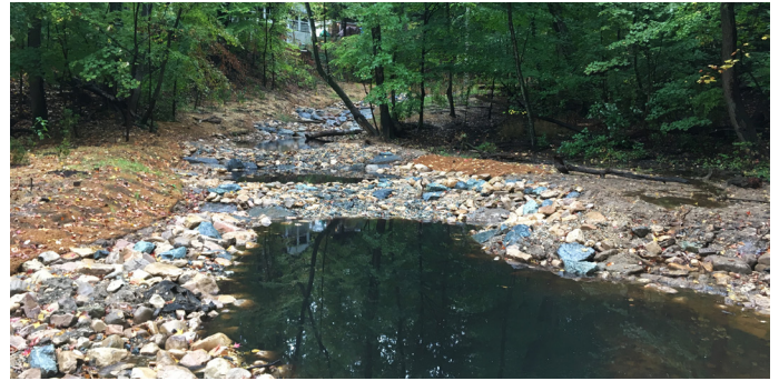
Step pools slow and retain stormwater
