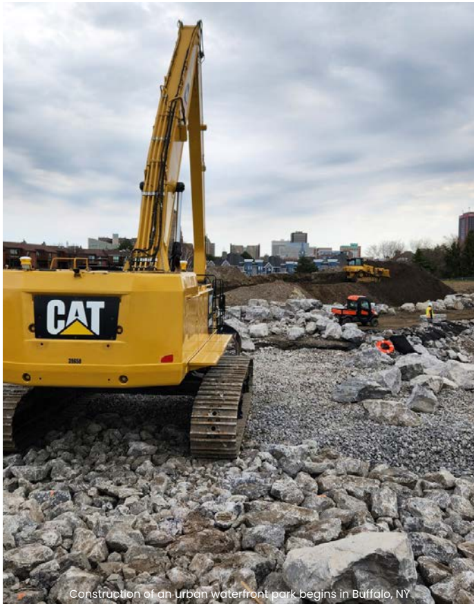
Construction of an urban waterfront park begins in Buffalo, NY
