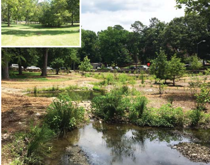
After restoration with inset of initial conditions
