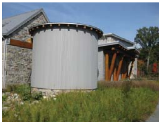
from top: Constructed wetland for wastewater treatment; Rainwater treatment system made visible for education; 10,000 gallon cistern for harvested rainwater
