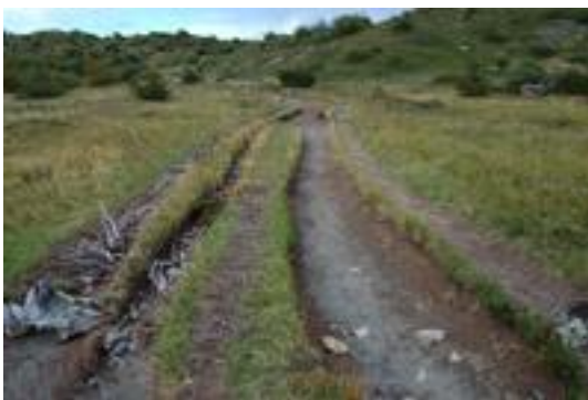
Before/after photos of a Conservation VIP trail restoration in Torres del Paine National Park in Chile. The new trail is constructed to shed water laterally rather than down the trail.
