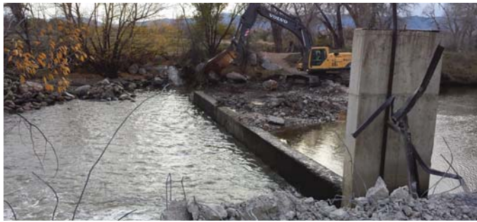
from top: River after dam removal; Removal of the dam
