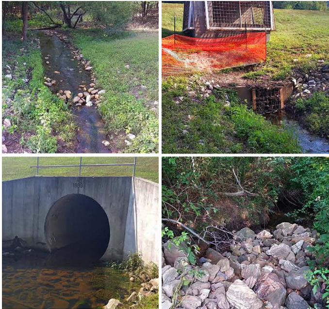
Mapping and photographs showing initial conditions— Regional Pond 341
