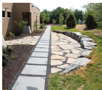
Clockwise from top: Stormplanter system filters pollutants; Permeable pavers absorb parking lot runoff; Repurposed library sidewalk, boulders from a local quarry, & native gardens form outdoor classroom
