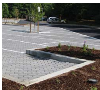
Clockwise from top: Stormplanter system filters pollutants; Permeable pavers absorb parking lot runoff; Repurposed library sidewalk, boulders from a local quarry, & native gardens form outdoor classroom
