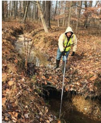
from top: Riffles with deep backwater pools immediately after construction; Assessing initial, severely eroded conditions
