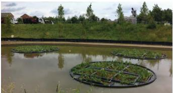
The Ponds at Potomac Yard are two existing stormwater management ponds that receive runoff from nearby development. These ponds ultimately discharge to the Potomac River, a tributary of the Chesapeake Bay. Biohabitats' ecologically engineered approach, designed in conjunction with Ambler Design, LLC, retrofitted the ponds to improve water quality
