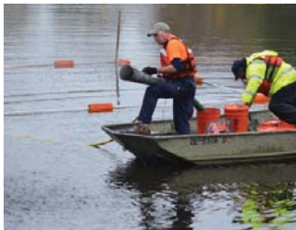
from top: Tidal wetland bench (left background) immediately after planting; Installation of sand utilizing a Telebelt®; Placement of SediMite™ from a boat using compressed air
