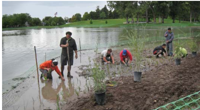
Installation of native wetland vegetation in newly constructed floating wetland (top) and newly created wetland benches (bottom)
