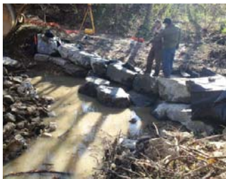
from top: After restoration; During construction; Severely eroded banks and collapsing retaining walls before construction
