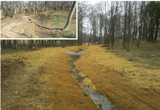
top: Mainstem channel banks after enhancement, before planting with initial conditions inset; above: Tributary reach after enhancement, before planting with initial conditions inset
