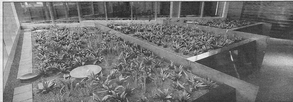
DJC file The Living Machine at the Port of Portland's headquarters uses wastewater treatment processes similar to those that will be used at Hassalo on Eighth.
