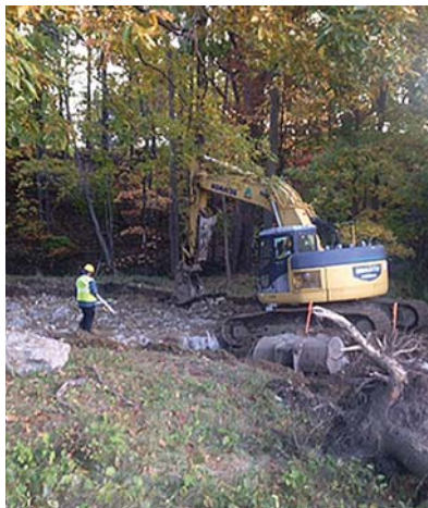
from top: Detail of conceptual design for area 1.2 on Euclid Creek; Installing a boulder riffle
