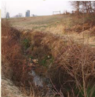
top: After restoration above: Initial conditions
